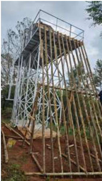
Scaffolding built to roll the tank from the ground to the top of the tower
