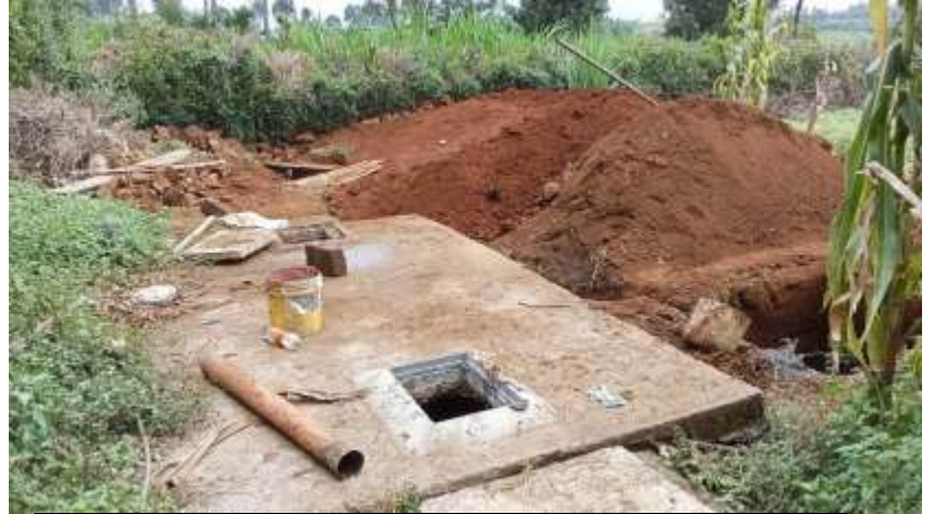
Emergency repairs on our seventeen year old septic system
